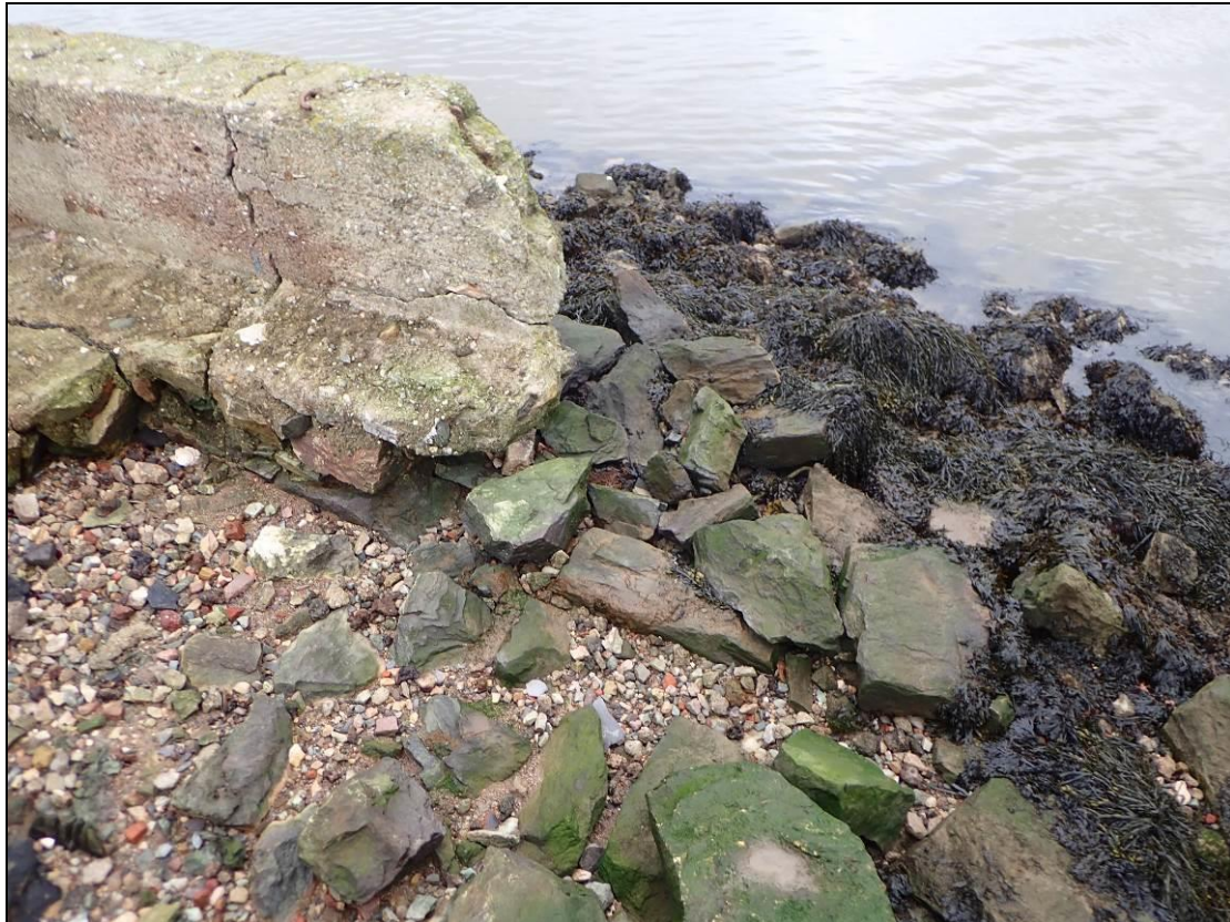
Plate 3: View showing the northeast corner of the Trinity Wharf boundary. The stonework below later concrete relates to the line to the older dockyard wall.
