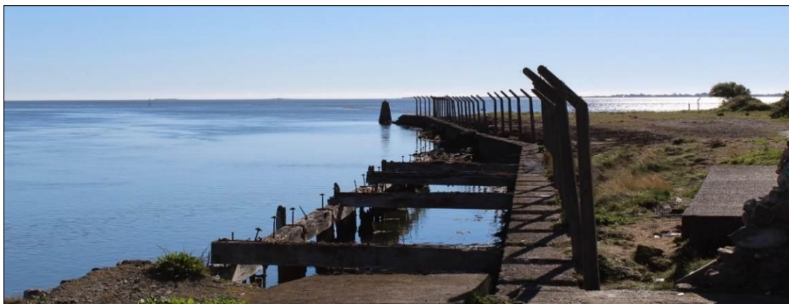
Plate 11.16 Wharf remnants along eastern edge
