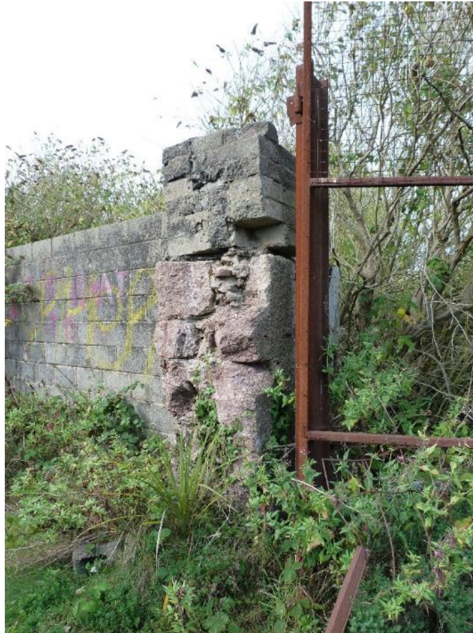
Plate 15.6 Gate pier to south of site
