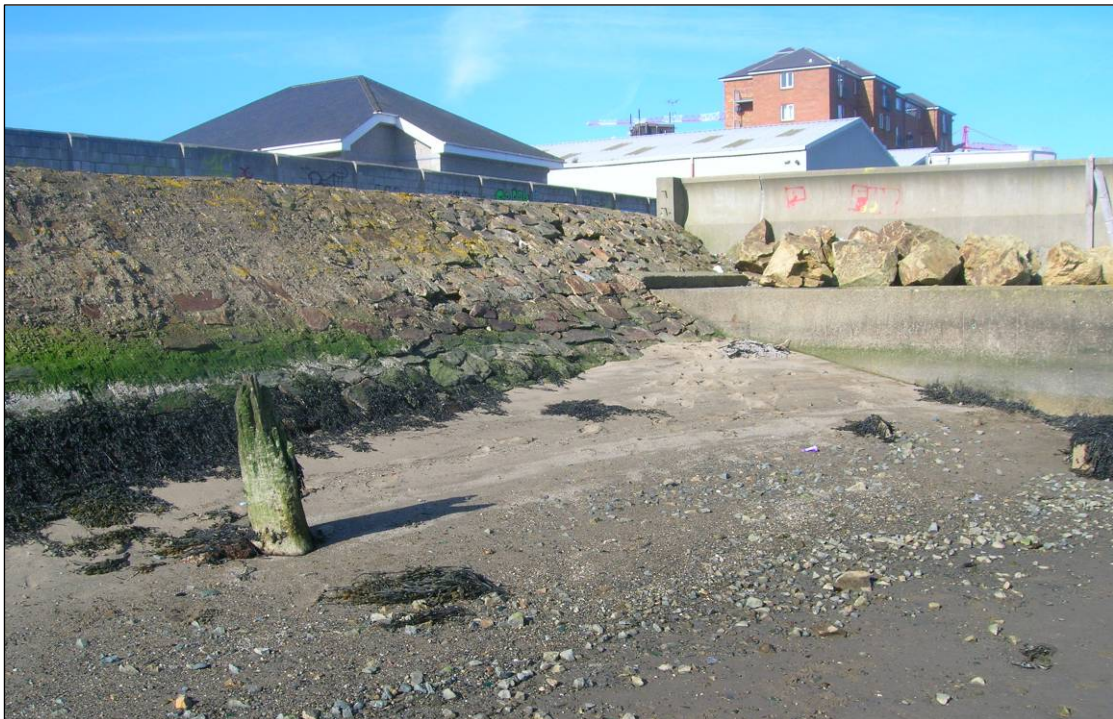
Plate 4: Foot of the railway embankment that defines the SW side of the development, where it is built onto by the newly reclaimed car park and quayside that runs north from here. The timber post in the foreground is an isolated instance and perhaps an old mooring post.
