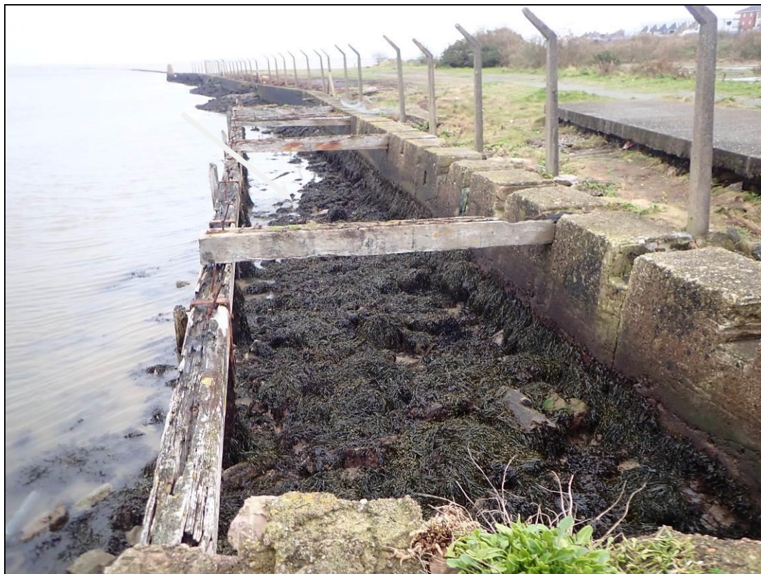
Plate 9: View looking south at the remains of a timber jetty that is integrated into the concrete copings of Trinity Wharf associated with the ironworking.
