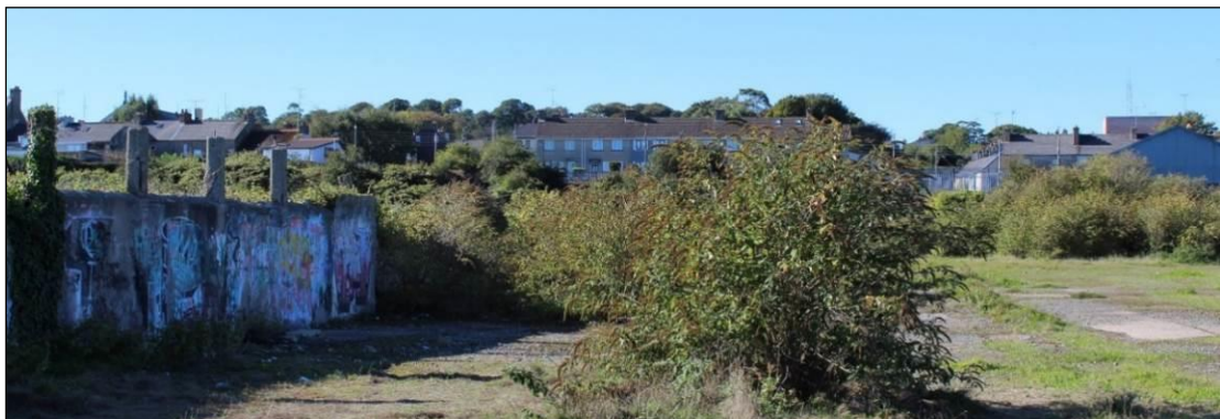
Plate 11.14 Walls, vegetation and areas of concrete on site
