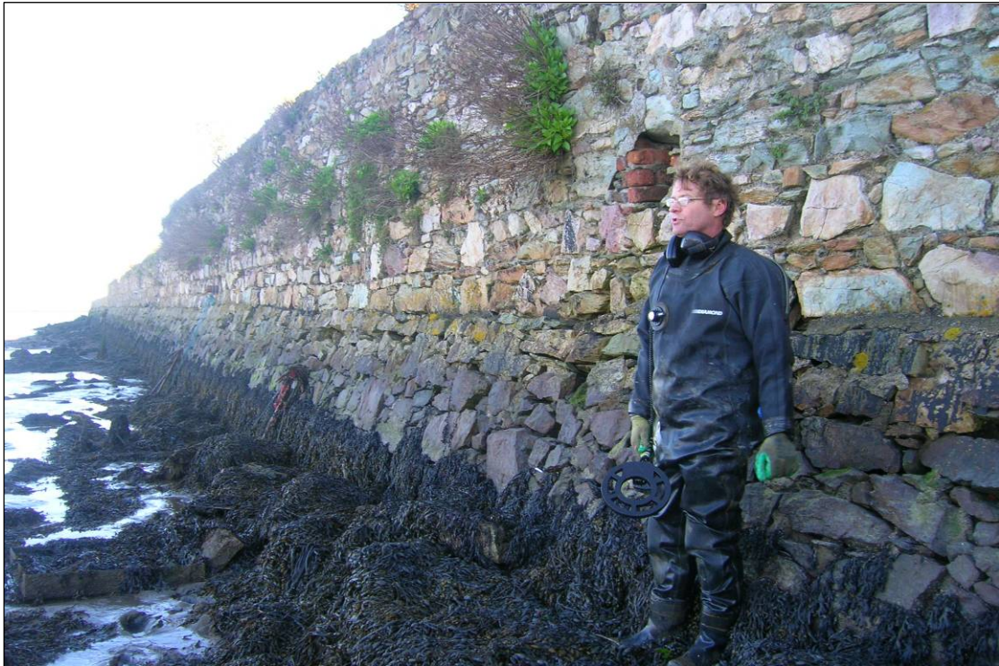
Plate 3: North-facing battered stone wall of former dock yard, at south end of proposed development site, with one example of the red-bricked drainage outflows indicated.
