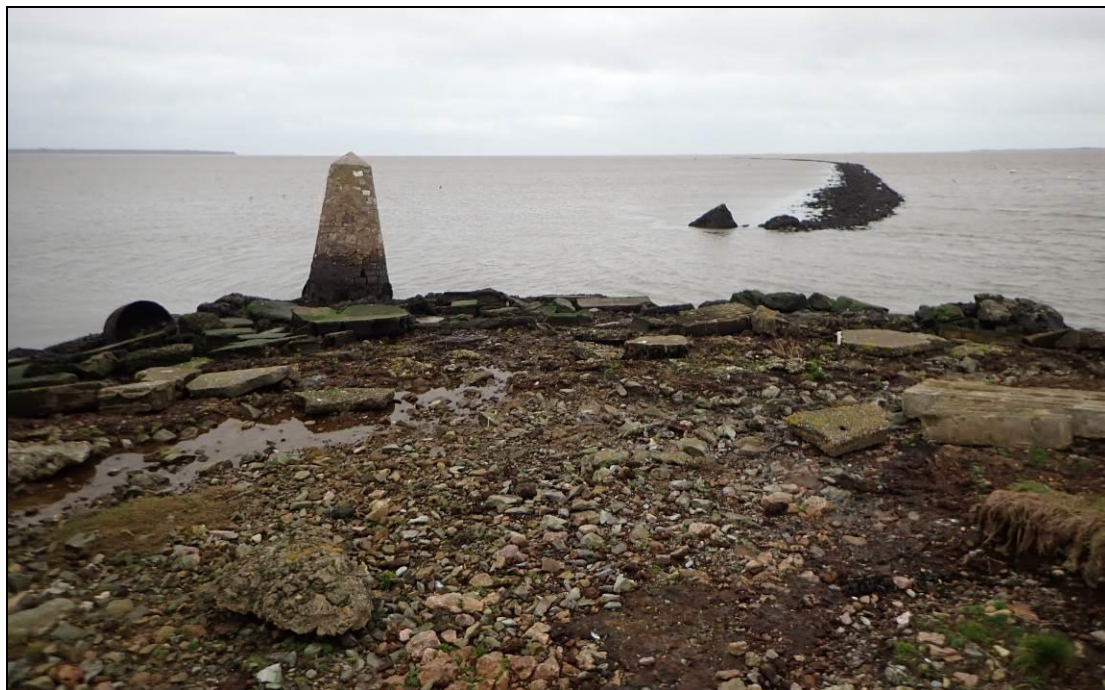
Plate 11: View looking southeast from Trinity Wharf at the stone-built navigation beacon that predates the wharf and served as part of the aids to safe passage into and out of Wexford Harbour. The breakwater is also visible.
