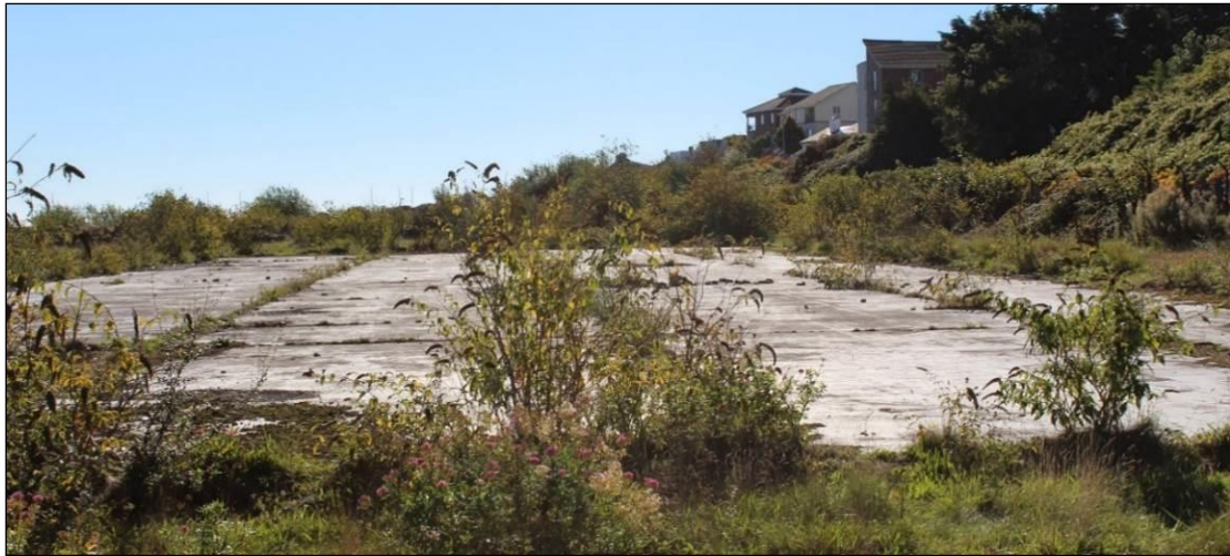
Plate 11.15 Concrete areas on site
