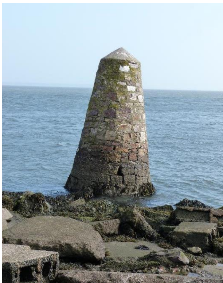
Plate 15.7 Beacon marking eastern corner of site
